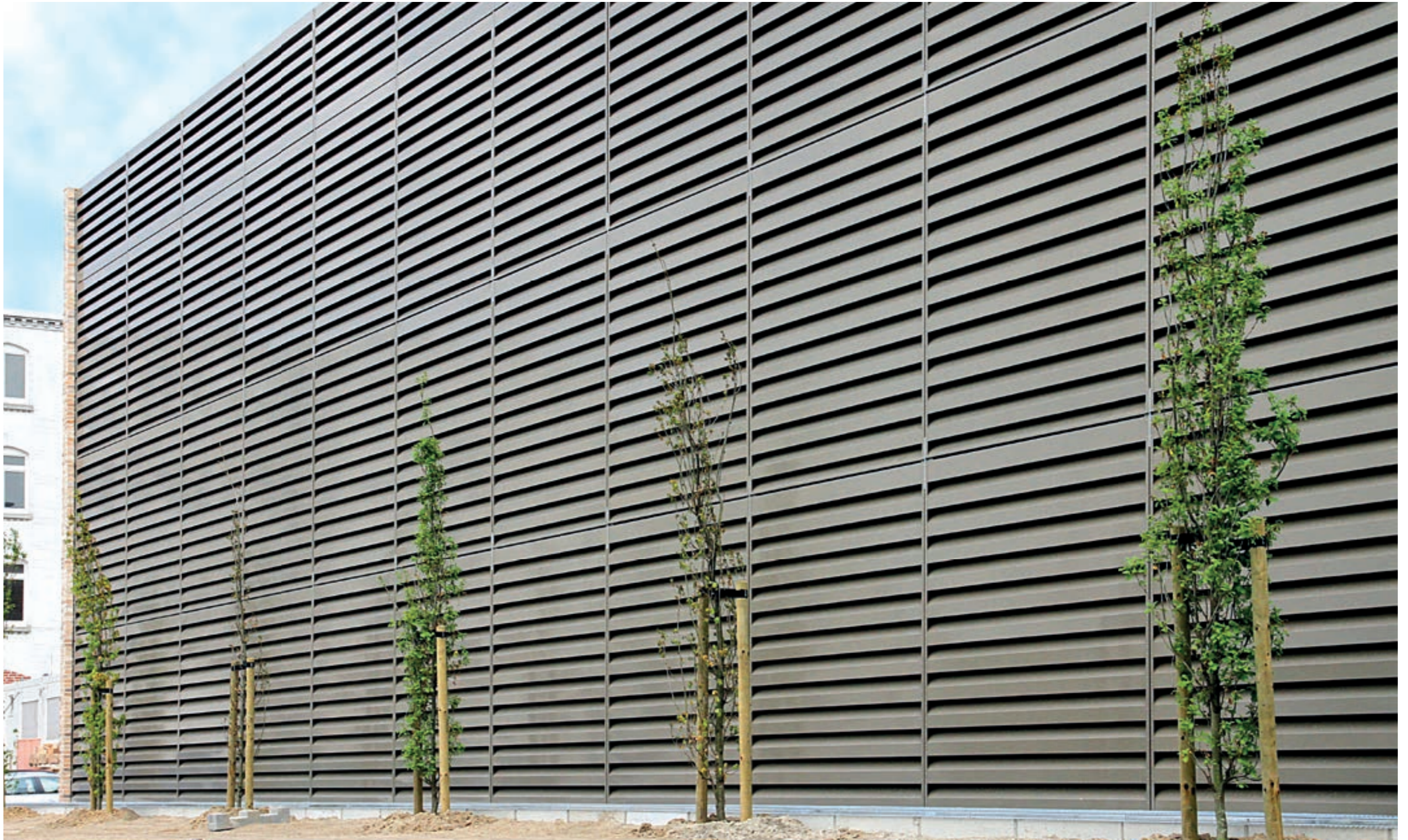
Parkhaus Lotter Straße in Osnabrück
